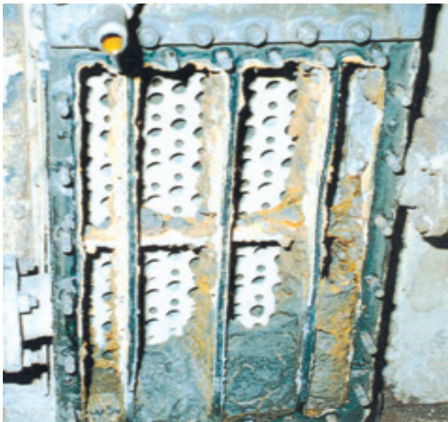
Fig. 12 — Heat exchanger after one year of service.
